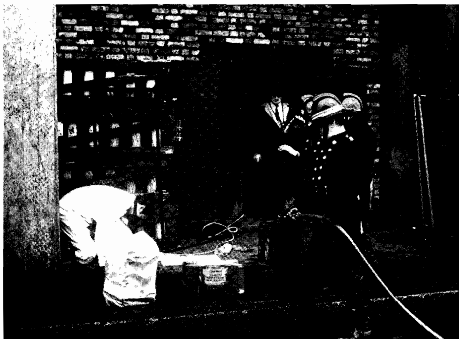
Fig. 3. Repacking hazardous material on location
